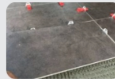
3 Place the other Tile over the other end of Tile Spacer
