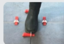
7 Simply Remove Wedges with a kick
