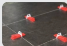
6 Let adhesive (Tile Glue / Cement) dry as recommended
