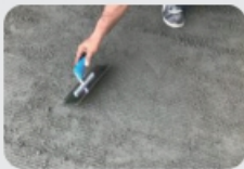
1 Apply Tile Glue / Cement
